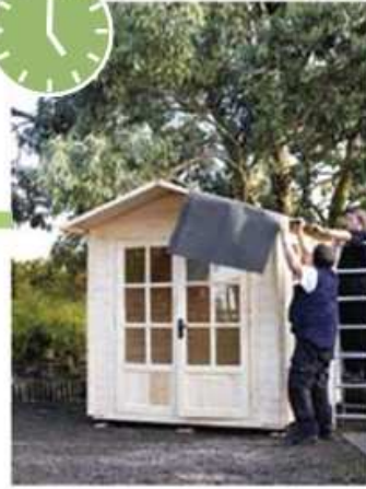
LAY FELT ROOF
